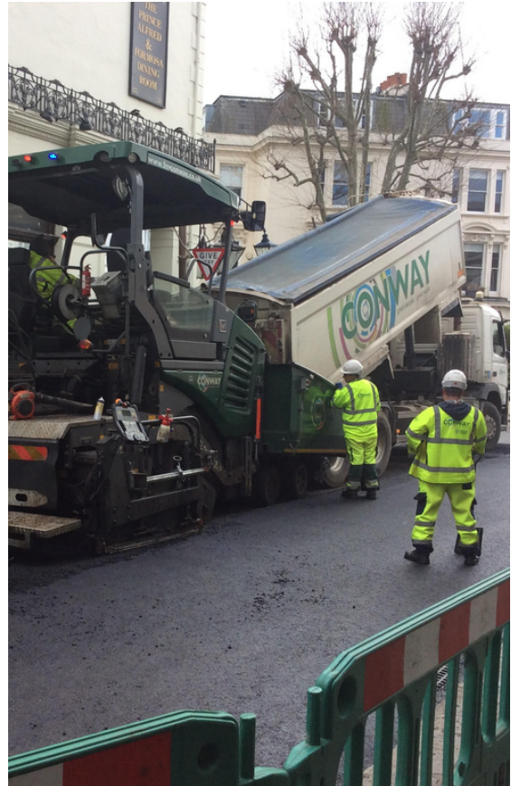
Carriageway resurfacing on Formosa St
