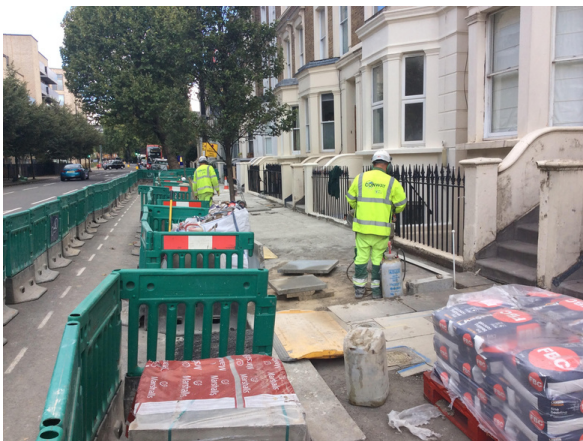
Footway renewal Kilburn Park Road
