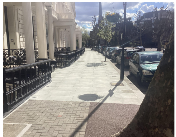
Brand new finished Warrington Crescent footway
