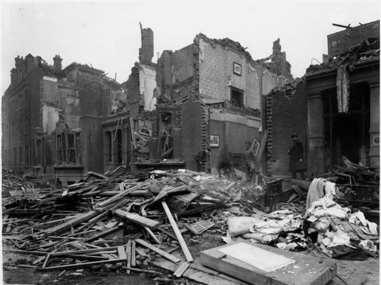
Above: Damage outside 61 to 65 Warrington Crescent following the Great Air Raid of 1918.
